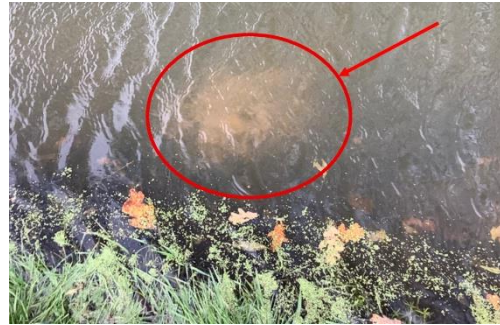
Figure 22. Piping Mastenbroek-IJssel (TAUW et al., 2024)
